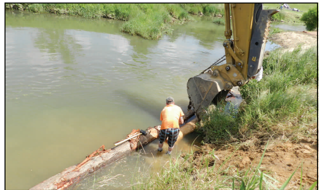
In Progress: log deflectors being placed in stream.
