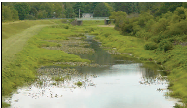
Before: Phase III improvements have not begun.
